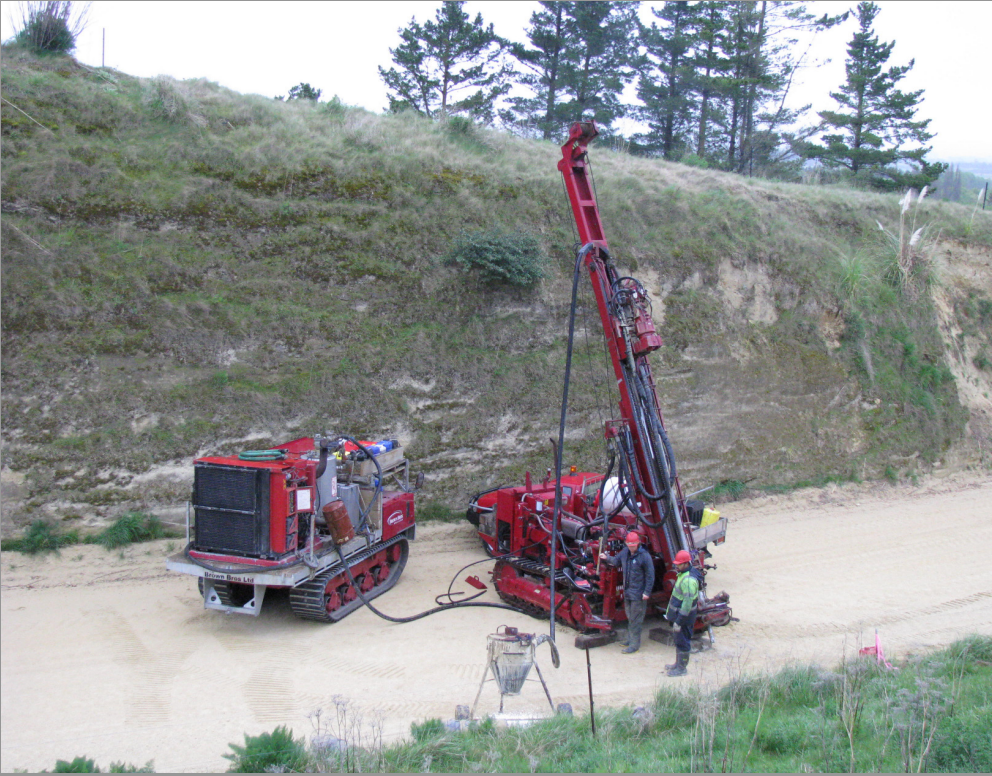
Rig 8 - Angle Hole Drilling - 3" Reverse Circulation Hammer
